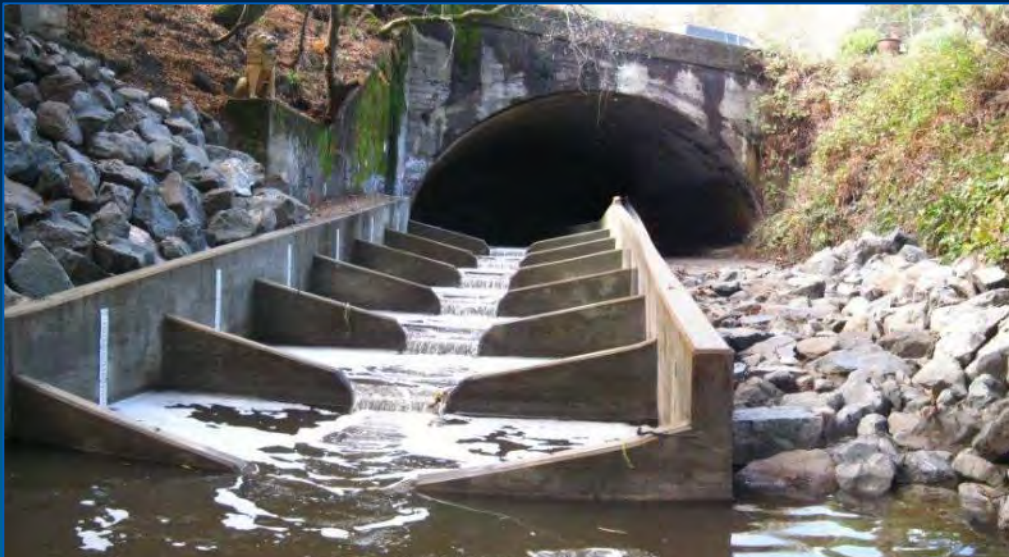
Partial Width Pool-and-Chute Fishway
