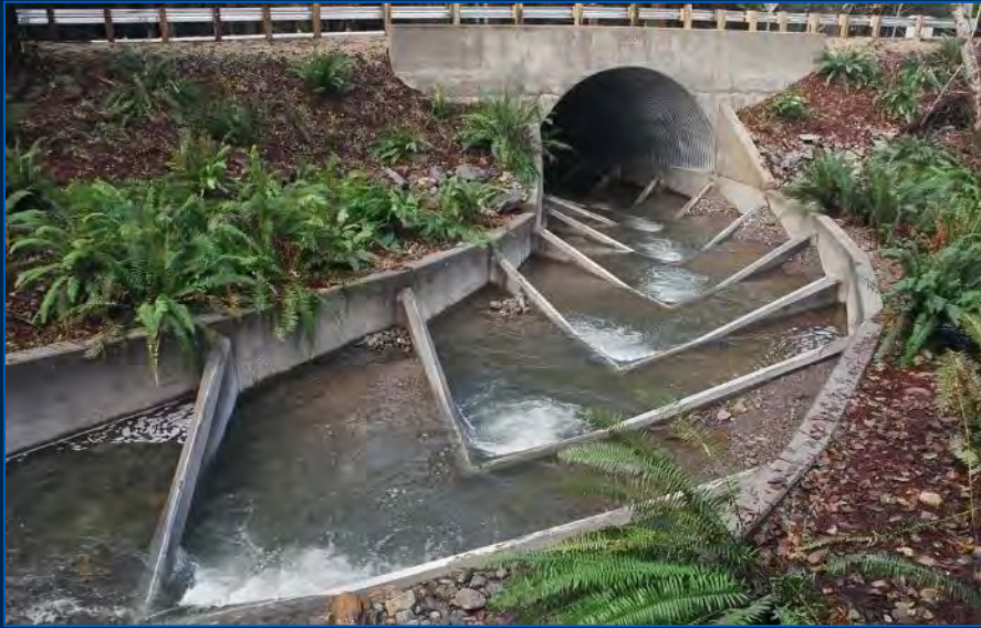
Full Width "Vortex" Pool-and-Chute Fishway
