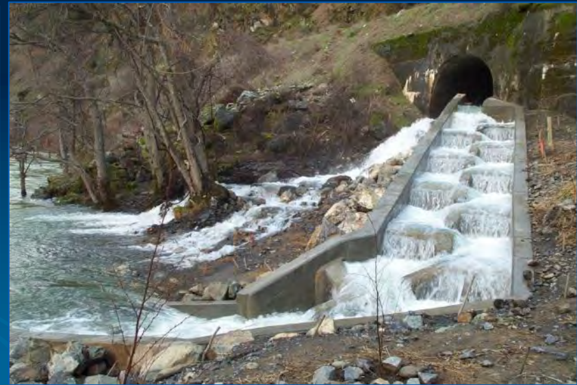
Bypass "Serpentine" Pool-and-Weir Fishway
