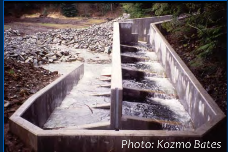
Bypass Pool-and-Weir Fishway
