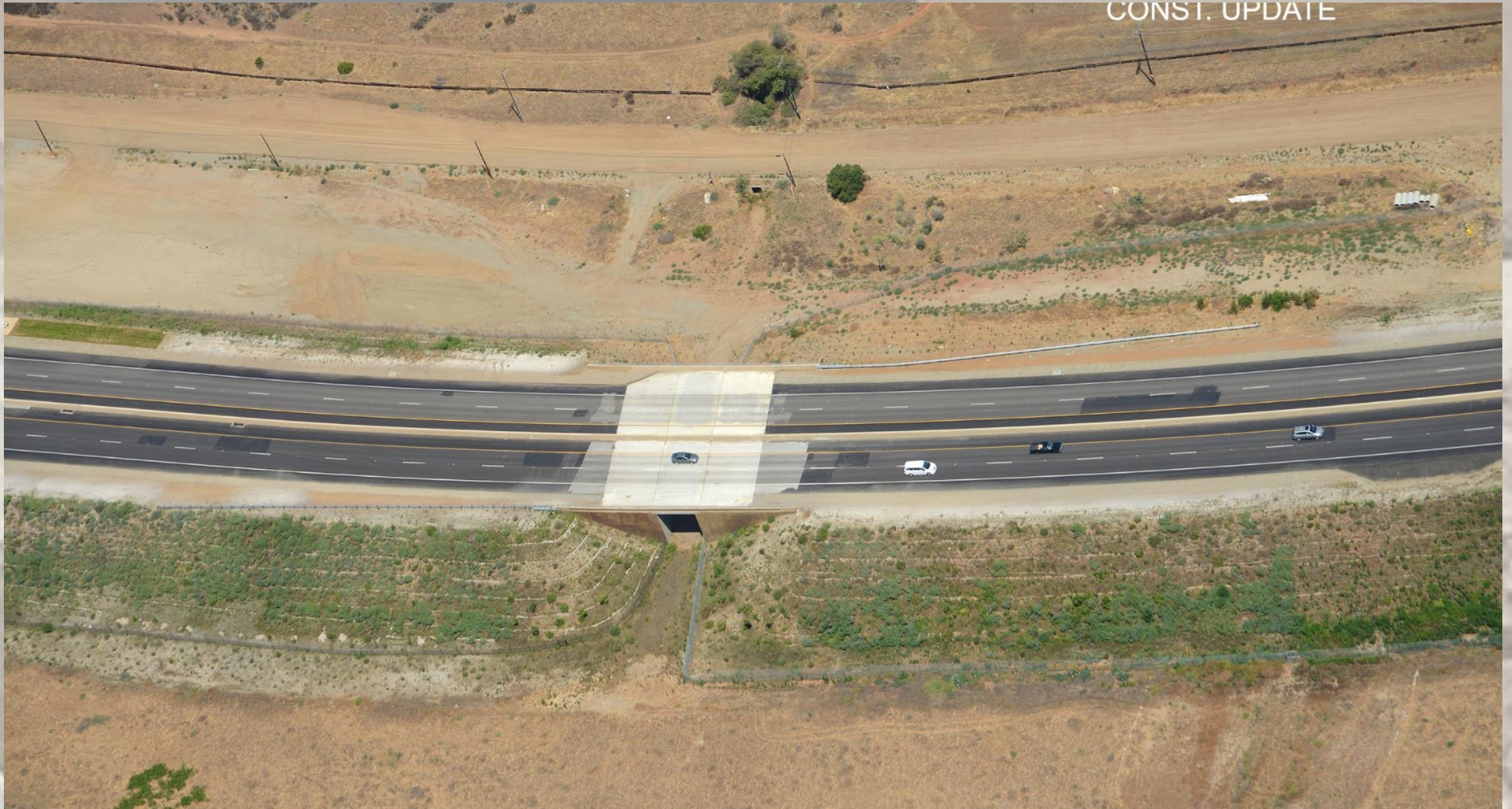
Aerial View of Completed Wildlife Crossing and Fencing at Via Montellano
