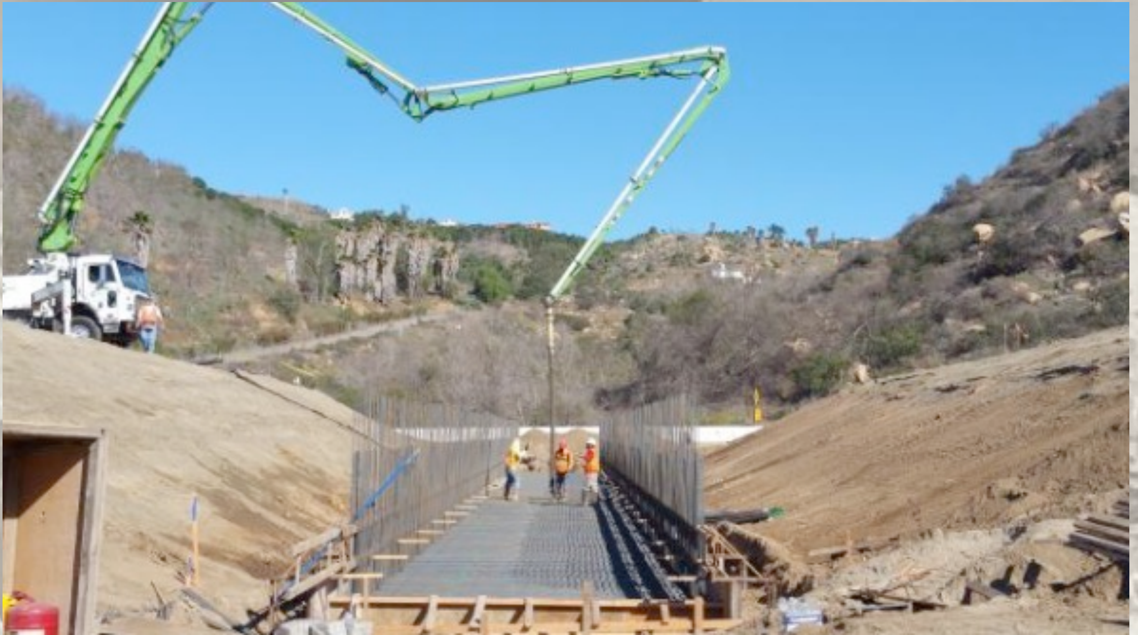
Wildlife Crossing Under Construction at Via Montellano
