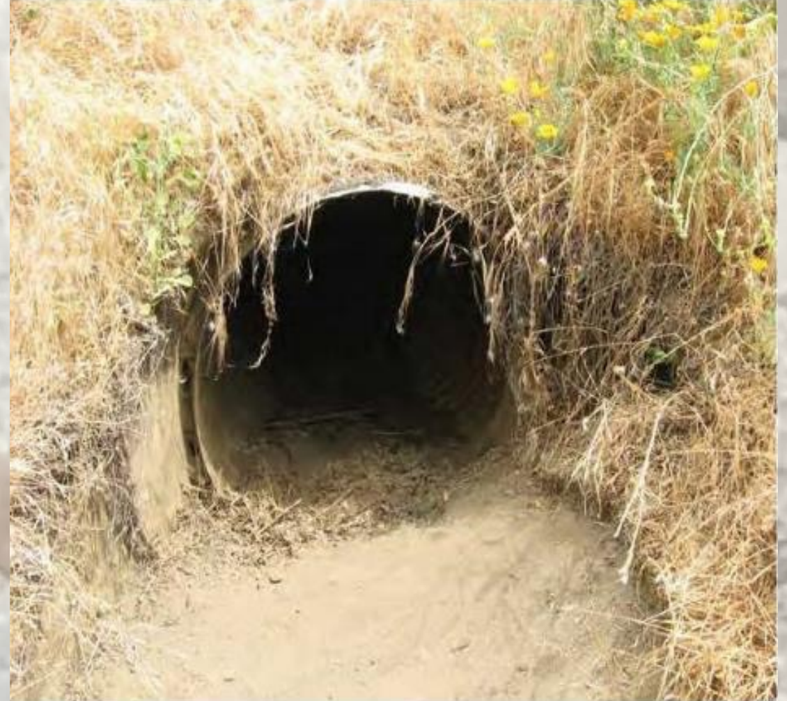
Pipe culverts at SR-76 and Gird Road
