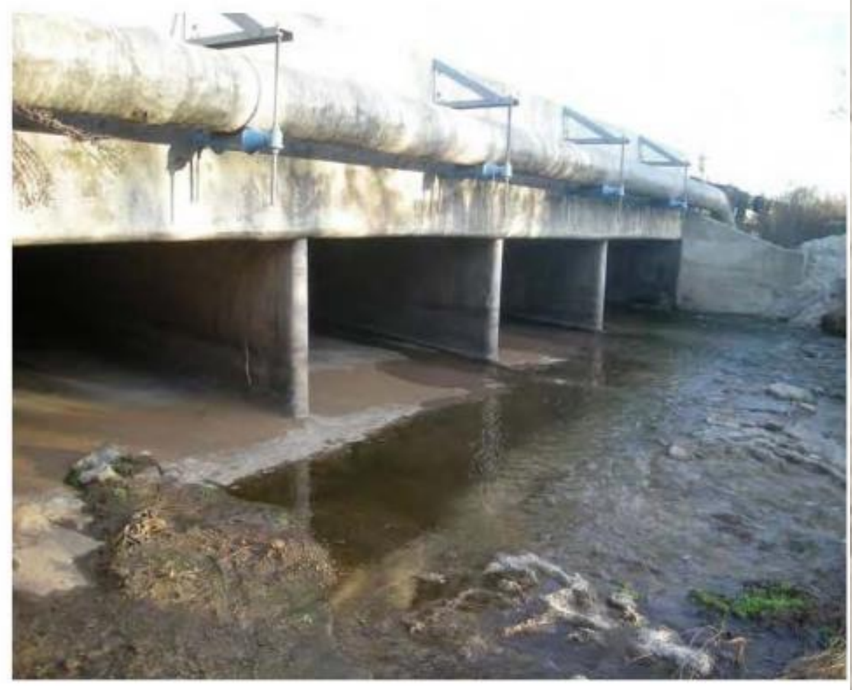
Ostrich Farm Creek Bridge
