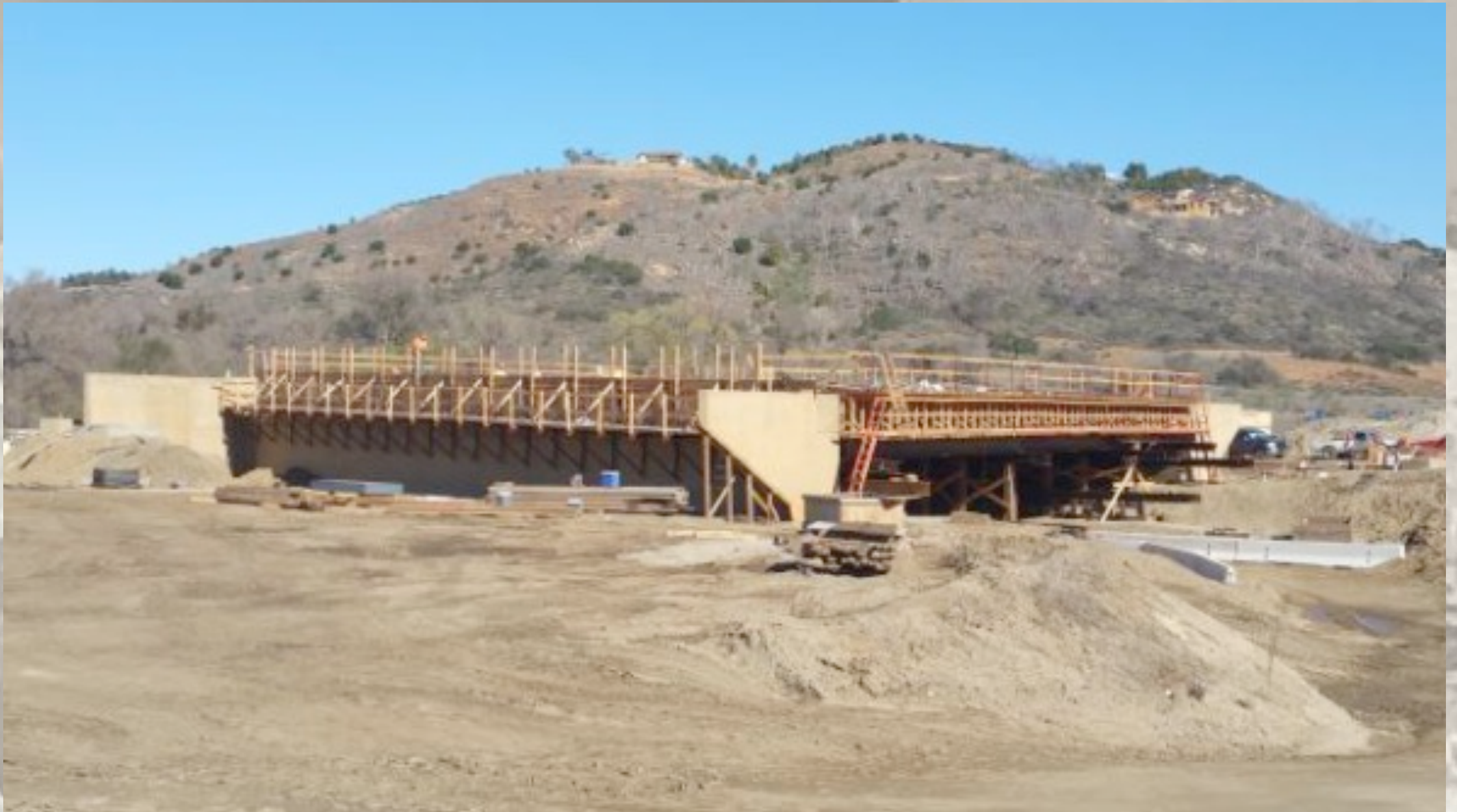
Live Oak Creek Bridge During Construction
