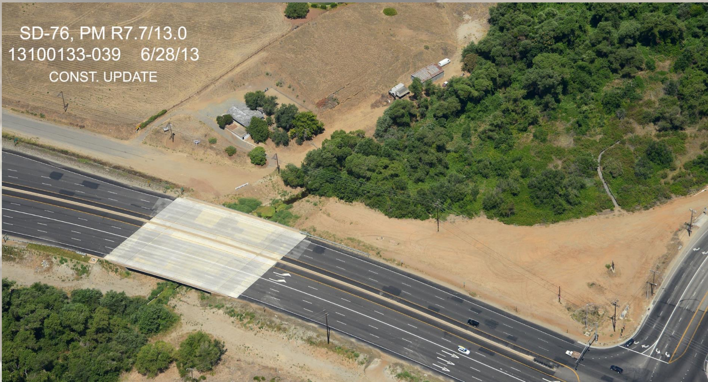
Ostrich Farm Creek Bridge Wildlife Crossing
