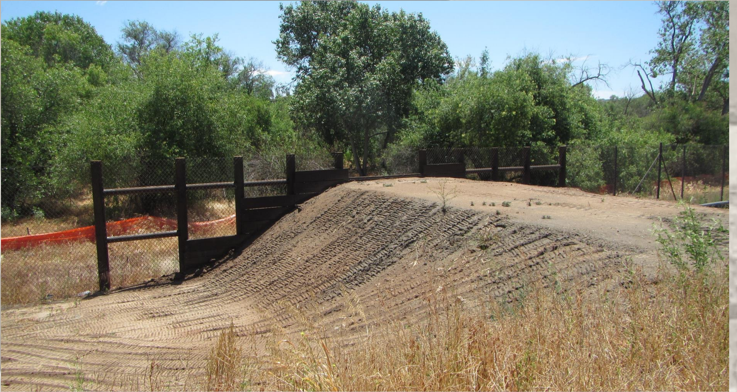
Completed Wildlife Escape Ramp
