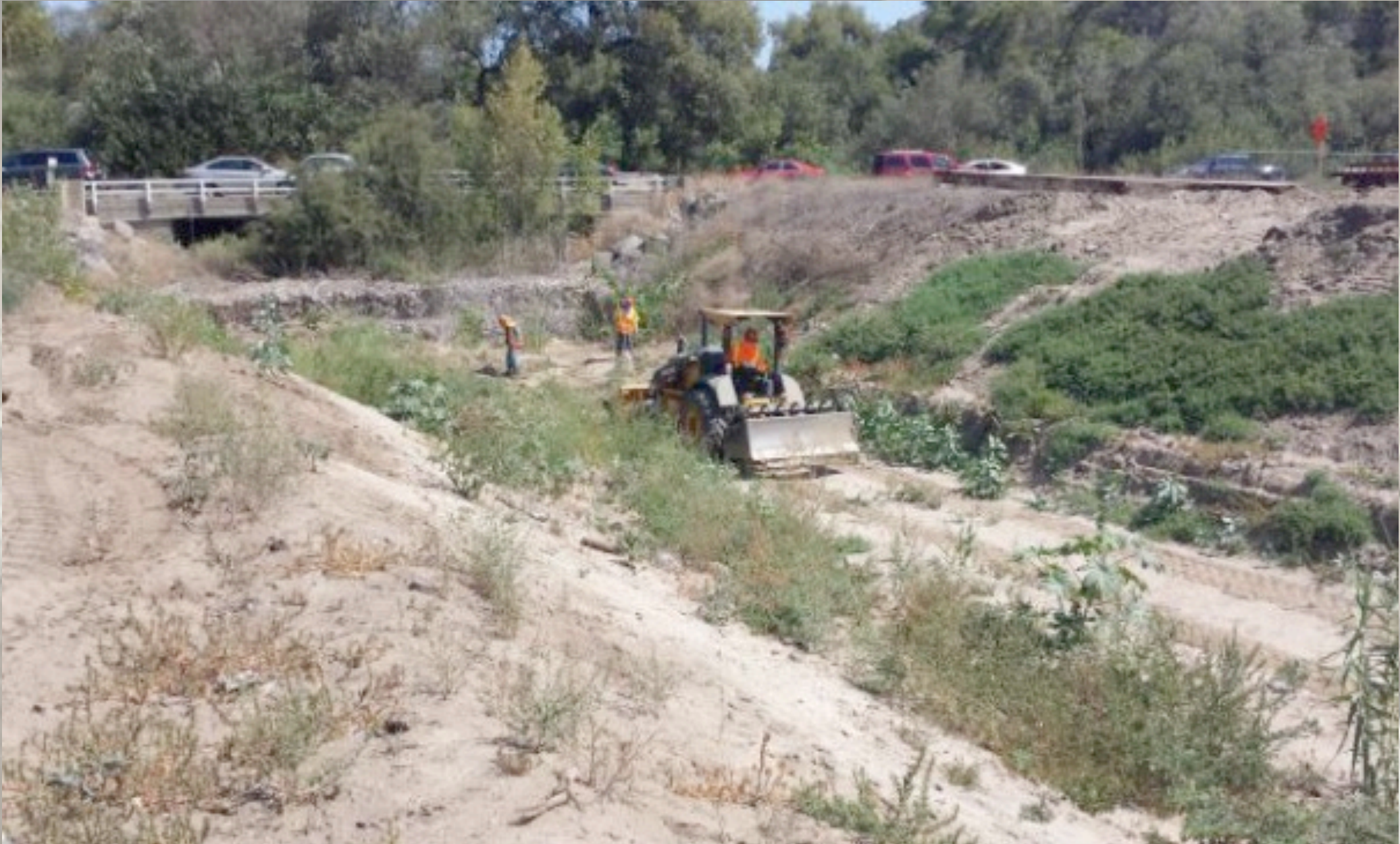
Bridge Construction Beginning at Live Oak Creek
