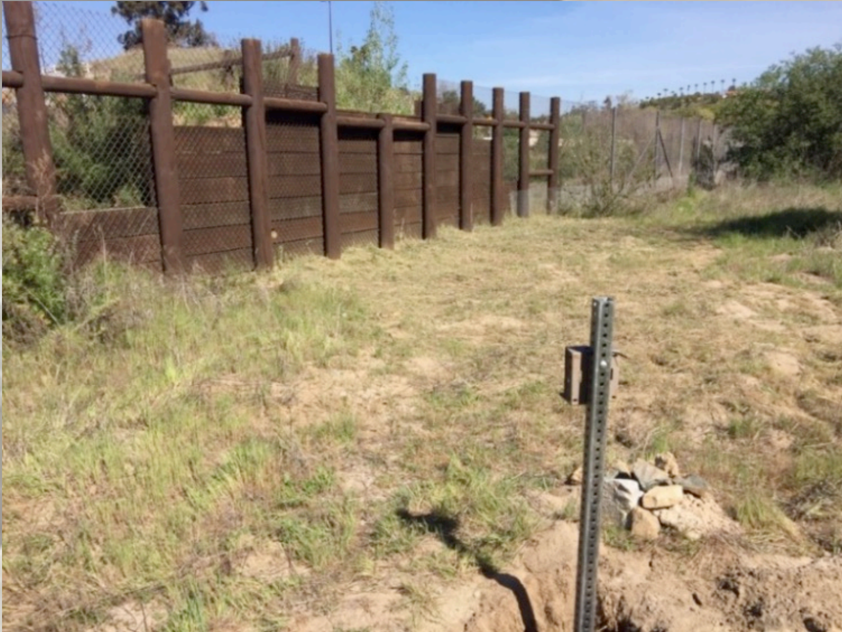
CAMERA STATION AT ESCAPE RAMP
