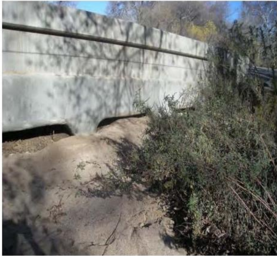
Box culvert at Flowerwood Lane
