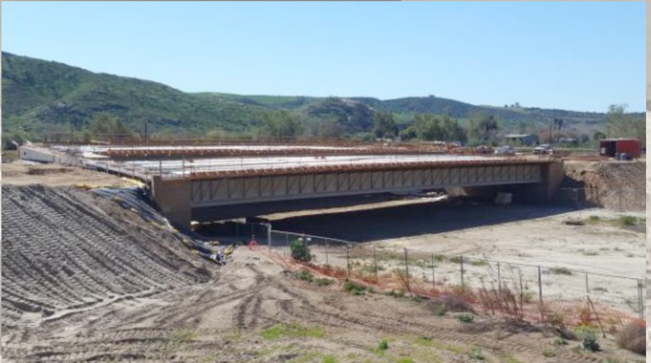
Bridge over the San Diego Regional Water Authority Pipeline
