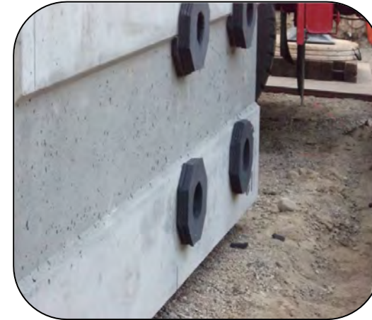
Post-tensioning ducts ran through abutment elements
