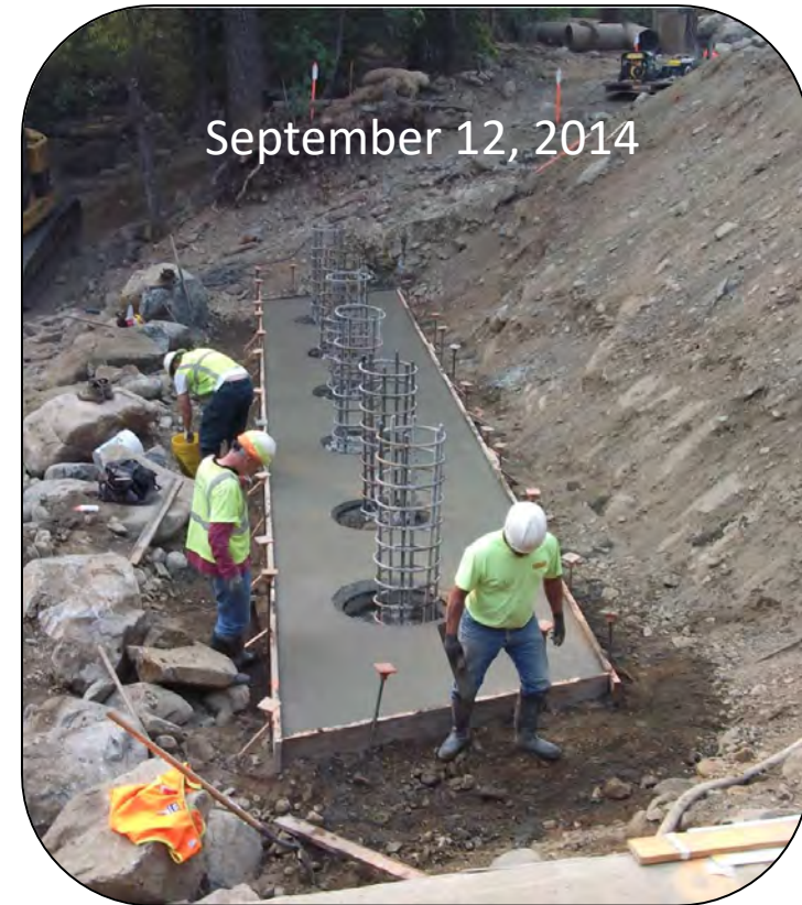
4 sac slurry for abutment bearing pad proved an effective leveling pad.
