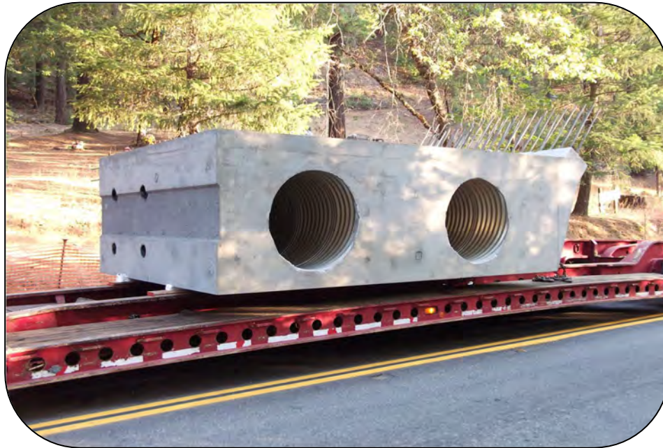
85 kip precast abutment elements (1 kip = 1,000 pounds)
