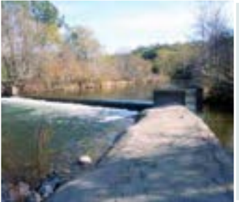
Deer Creek Irrigation Dam
