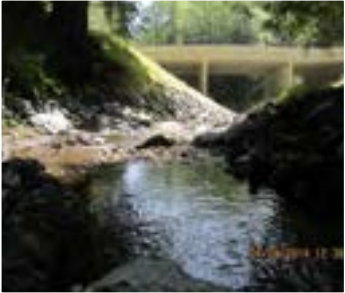
Dunn Creek Bridge
