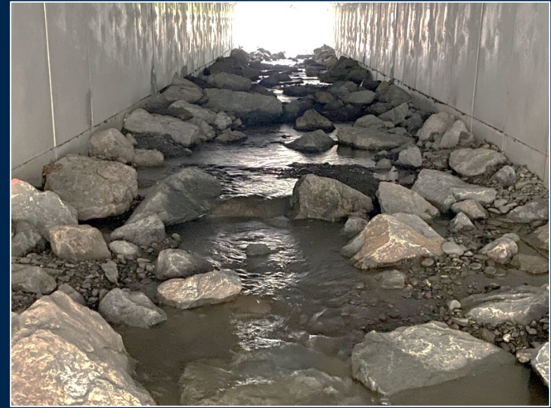
Example of a “roughened channel” grade control in a box culvert
