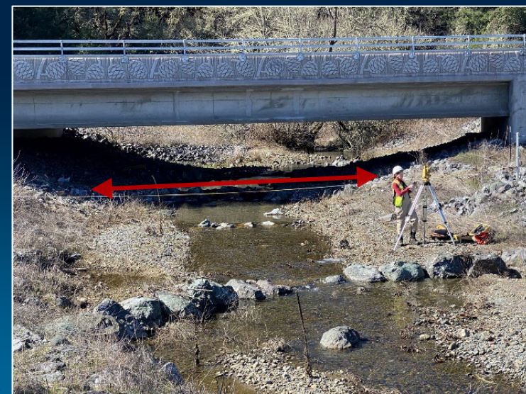
Downstream Bridge Face
