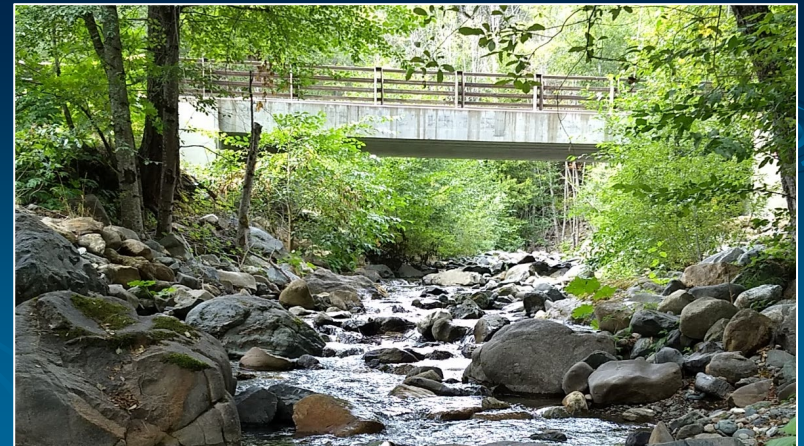
Fort Goff Bridge Channel
