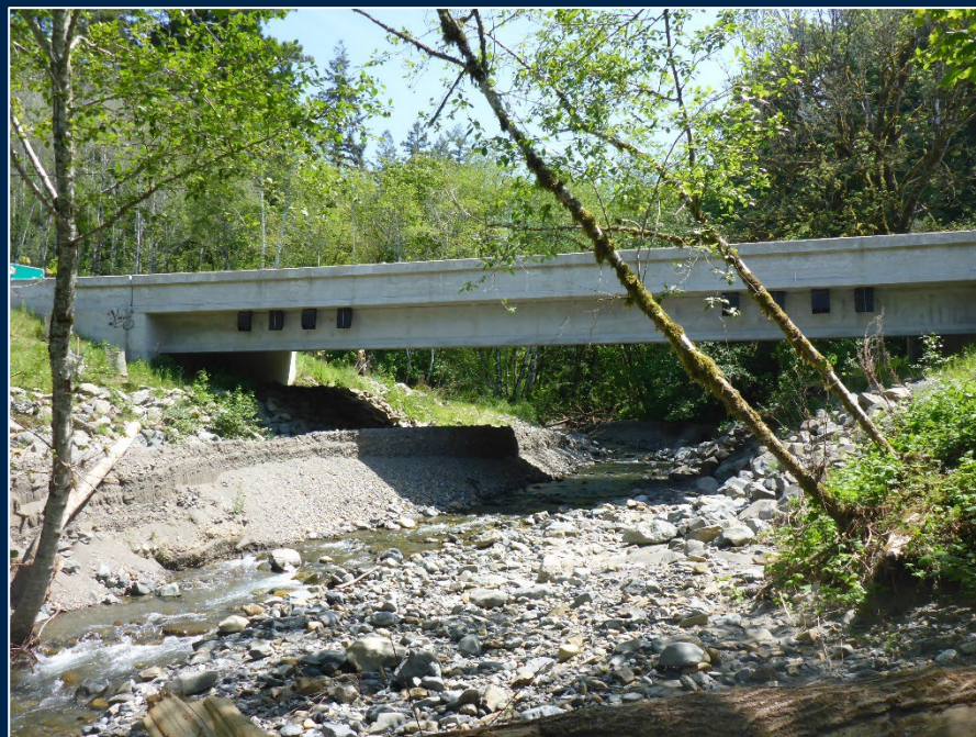
Little Mill Creek Full-Span Bridge
