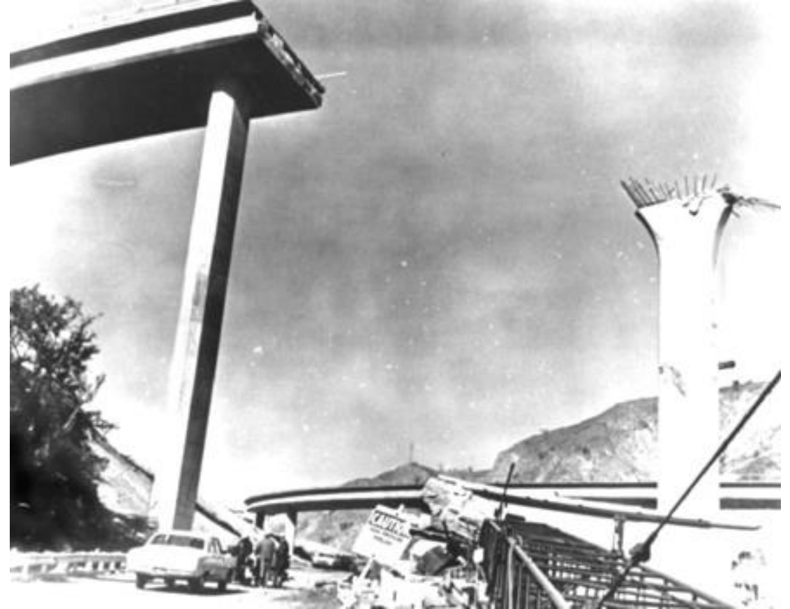
1971 San Fernando Earthquake, Magnitude = 6.5
