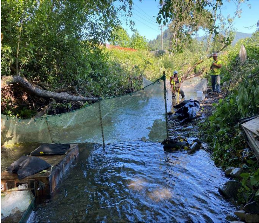
Install double block net
