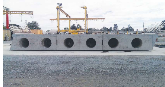
Preassembly of abutment elements at the fabricating yard ensured fit up with piles and tie rod ducts in the field.
