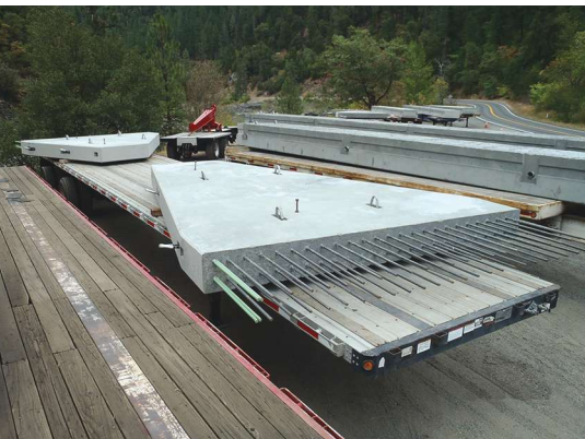
Precast concrete elements at the jobsite ready for quick assembly.
