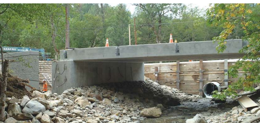
Precast concrete elements are connected by grouted keyways, post-tensioned tie rods, and closure placements.
